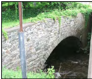
Stone Arch Bridge
