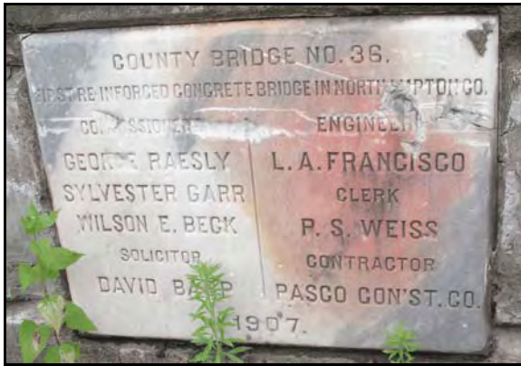
Route 611/Jacoby Creek Bridge
