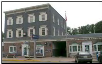
PNC Bank and Post Office
